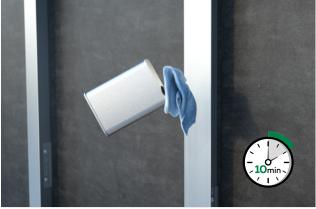
Cleaning the sub-frames with Innotec<sup>®</sup> Multisol Project – Note time to ensure a waiting time of 10 minutes before the next step at the sub-frame.
