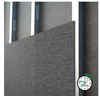
Attach the panel to the sub-frames within 10 minutes after application of the adhesive, and press firmly. Ensure to keep the minimum distance of 8mm between each panel and use a level device to ensure proper alignment.
