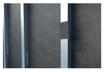
3. Prepare the aluminum sub-frame by using a sanding fleece for cleaning.
