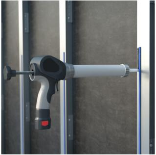
Apply Innotec<sup>®</sup> Adheseal Project adhesive onto the sub-frame with the accu gun. Ensure a proper positioning and share of the tape and adhesive. Leave 10 mm distance between the fixation tape and the side of the sub-frame.
