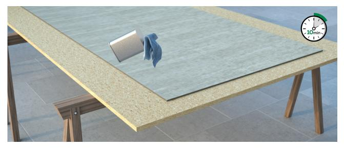
1. Mark the distance of the sub-frames and clean the areas of the backside of the Hardie<sup>®</sup> Panel where it will be glued – Note time to ensure a waiting time of 10 minutes before applying the primer.
