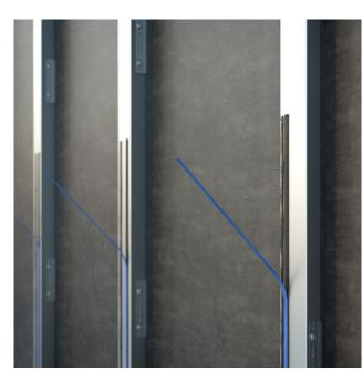
7. Remove the protection layer from the tape.
